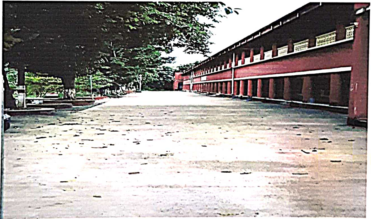
Nayagarh Autonomous College Main Building
